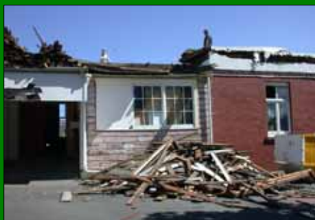
St Joseph's Church deconstruction in Wellington
