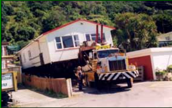
House leaving site on the back of a truck 1
