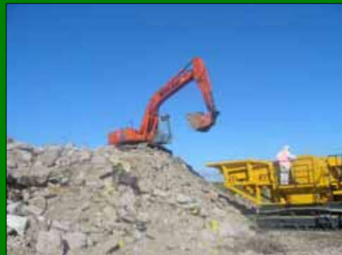
Crane loading concrete crusher 3
