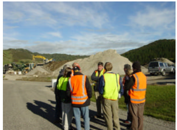
Peter Fredricsen talks about concrete crushing
