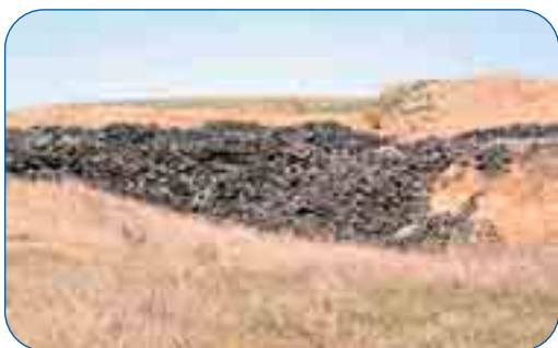
Tyre trench in Canberra which is covered regularly and divided into cells
