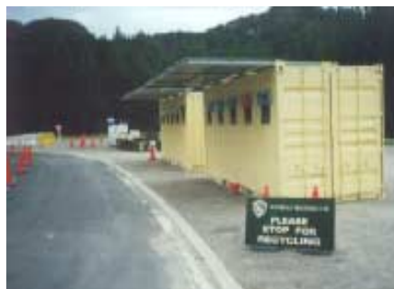
Sorting Facility at Rotorua Landfill
